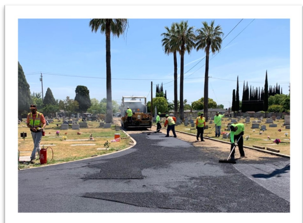
Finishing touches on the newly-laid road!
